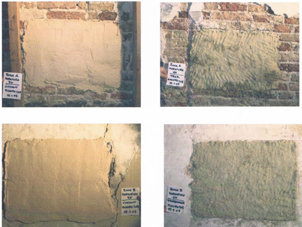
Figure 2 - The poultrices on the two types of substrate (bricks at the top - Marmorino below): Westox Cocoon on left and Arbocell + Sepiolite on the right
